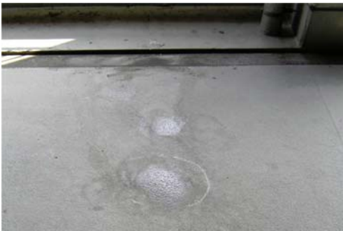
Photo 1-3: Water Filling Directly below; Before Construction Work, 20 Hours Later
